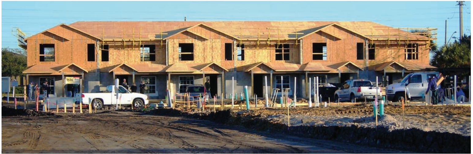
The 1st building of 10 in Habitat Orlando's first town home community"
